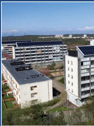
The renovation of the Gårdsten suburb of Göteborg won the UN World Habitat Award, 2005. Significant energy savings have been achieved through effective energy planning in this landmark development.
